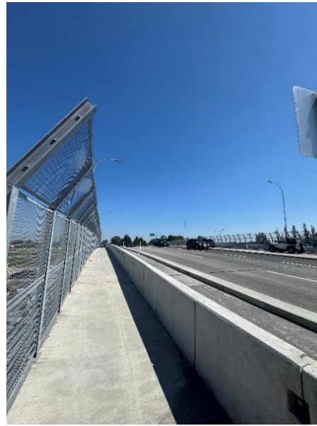
Figure 2: Overpass safety barrier, sidewalk and multi-use path looking east.
