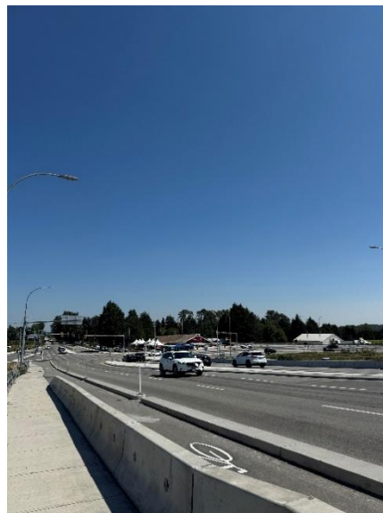
Figure 3: Eastern side of the overpass showing all five lanes, sidewalk and multi-use path.
