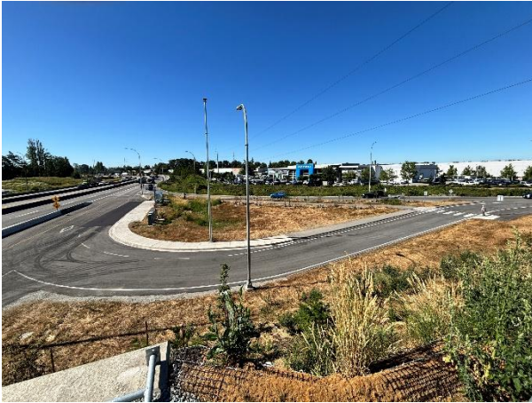
Figure 1: Southbound transit hook ramp onto Highway 99 with landscaping.
