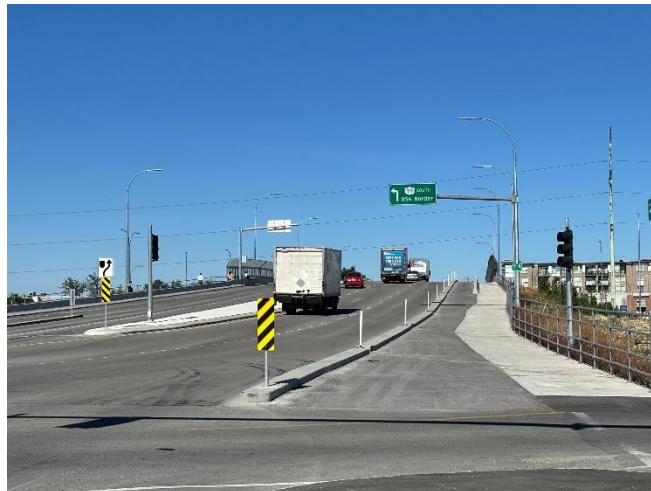
Figure 1: Sidewalk and cycle lane on east side of overpass.
