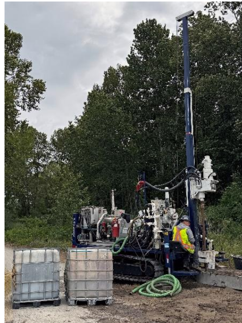
Figure 3: Geotechnical investigations for casting basin design and construction on Deas Island.
