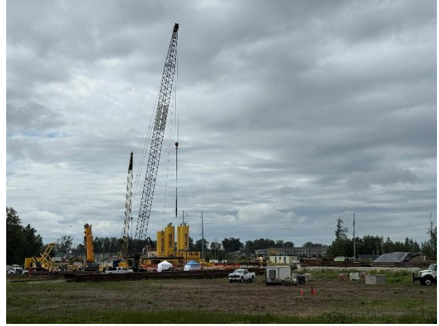
Figure 2: Stone column densification trial works on Deas Island.
