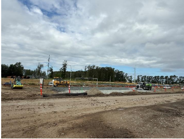
Figure 1: Construction of working platform for casting basin works on Deas Island.
