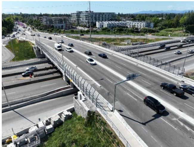
Figure 1: Drone image of the new five-lane overpass looking west.
