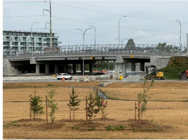
Figure 2: Landscaping and drainage channels in the northbound loop ramp looking northwest.
