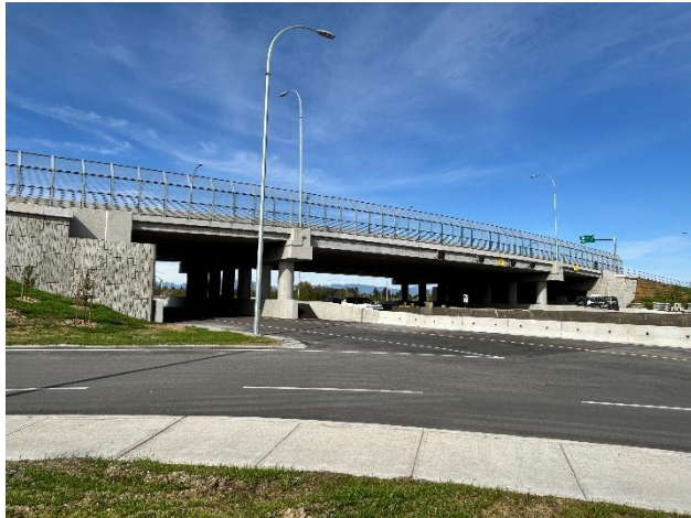
Figure 1: Completed overpass with new landscaping looking northeast.
