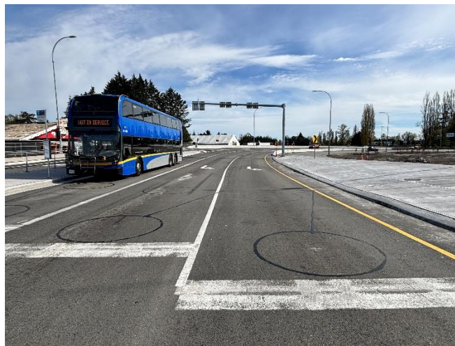
Figure 3: Transit lane and dual left-turn lanes on the northbound off-ramp.
