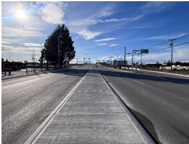
Figure 3: Steveston Highway concrete median on the east side of the new overpass, facing west.
