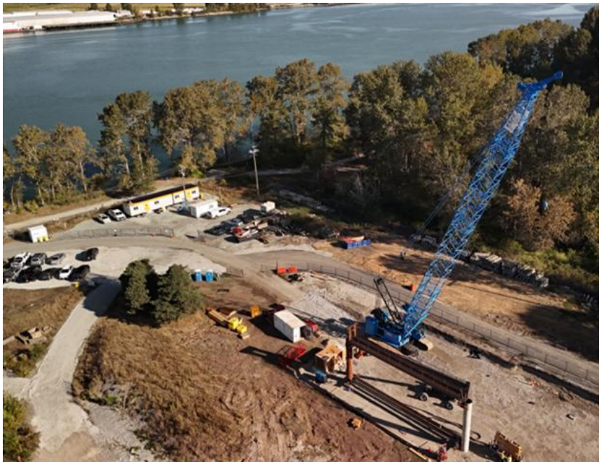
Figure 2: Geotechnical investigations begin on Deas Island within the Ministry's right-of-way. (Sept. 25, 2025)
