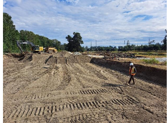
Figure 2: Site preparations underway on Deas Island for geotechnical work within the Ministry's right-of-way. (August 2025)
