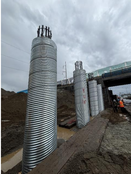
Figure 1: Southwest abutment piles in corrugated steel sleeves.
