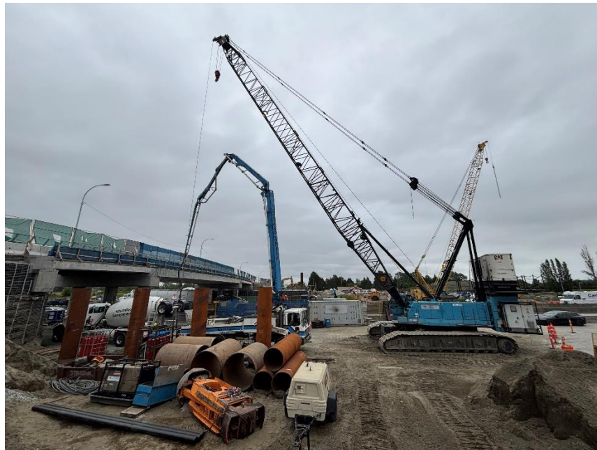
Figure 3: Pouring concrete for the southwest pier piles.
