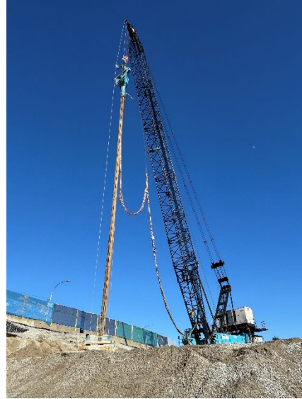
Figure 2: Heavy lift crane used for Phase 2 stone column work in the southeast quadrant.
