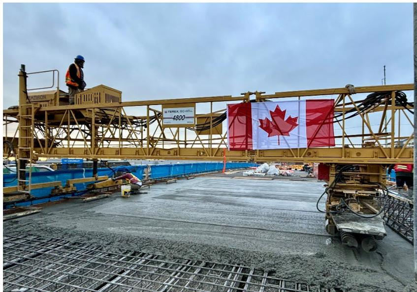
Figure 3: A paver machine placing and smoothing concrete during Phase 1 overpass deck pour.
