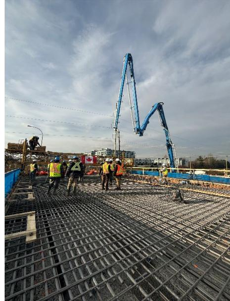
Figure 2: A concrete pump truck boom in place for west side Phase 1 overpass deck pour.
