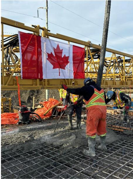
Figure 1: Crew members pumping and vibrating concrete for the west end of the Phase 1 overpass deck.
