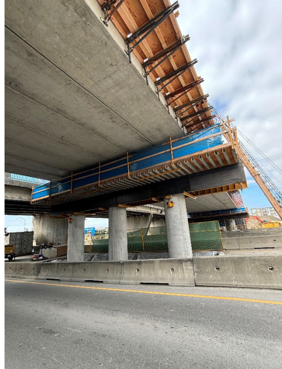
Image 2: All seven east side end-span girders in place.
