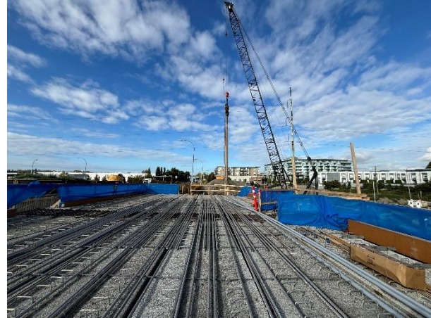
Figure 2: Preparation for rebar placement on the Phase 1 overpass deck underway.
