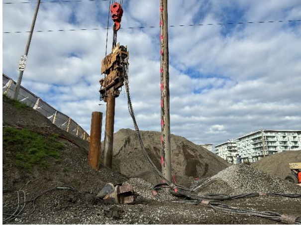
Figure 1: Impact hammer installing stone columns in the northwest quadrant.
