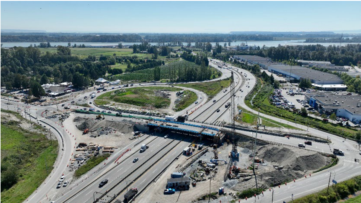
Image 1: Drone image facing south of the full Steveston Interchange Project site
