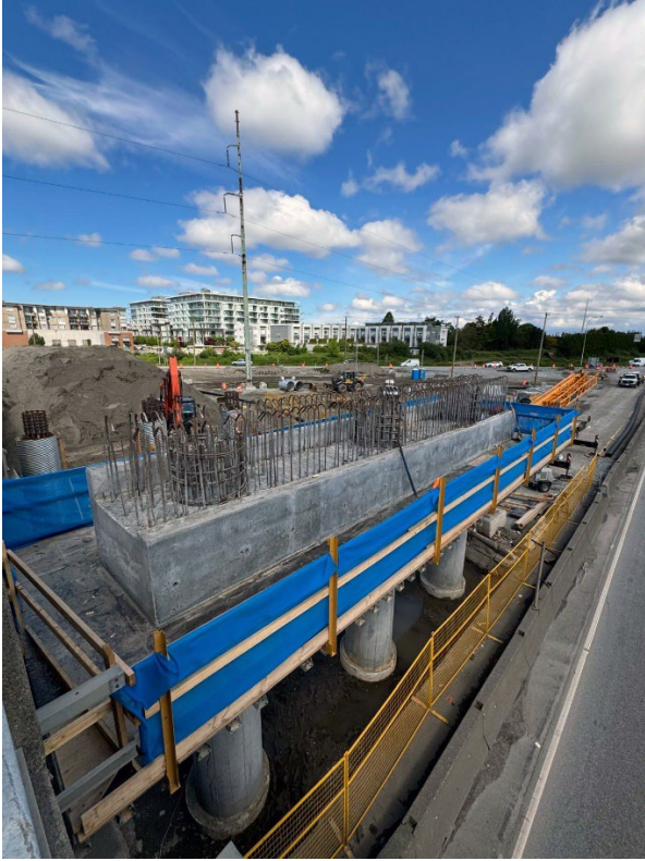
Image 2: Northwest pier cap with formwork removed
