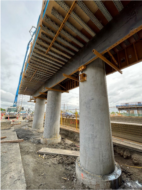
Image 1: Elevated work platform for pier cap construction in northwest quadrant
