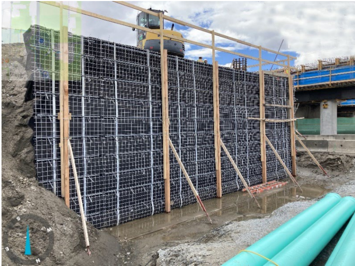
Image 3: Preparing northeast abutment for retaining wall panel installation
