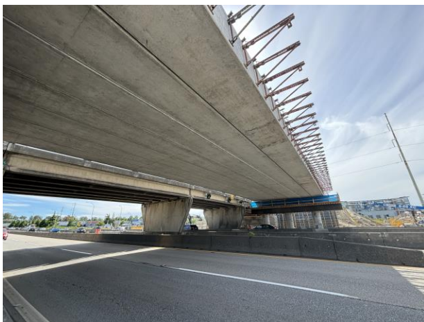
Newly installed Phase 1 girders spanning Highway 99.
