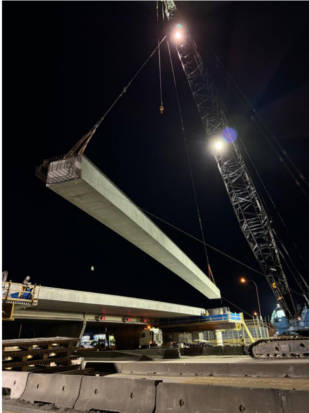
Heavy-lift crane hoisting a 35-metre, 50-tonne girder.
