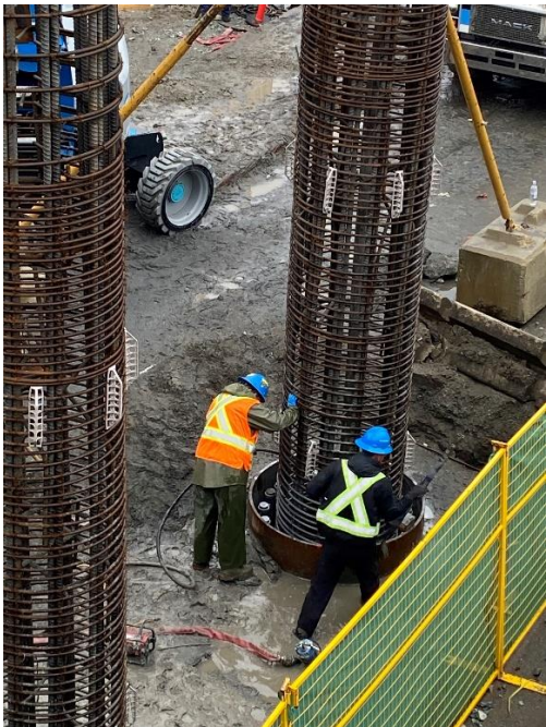
Image 3: Workers inspecting base of pier column cage
