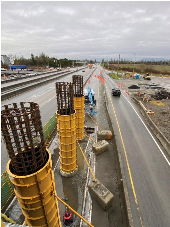
Image 2: Pier column formwork, northeast quadrant
