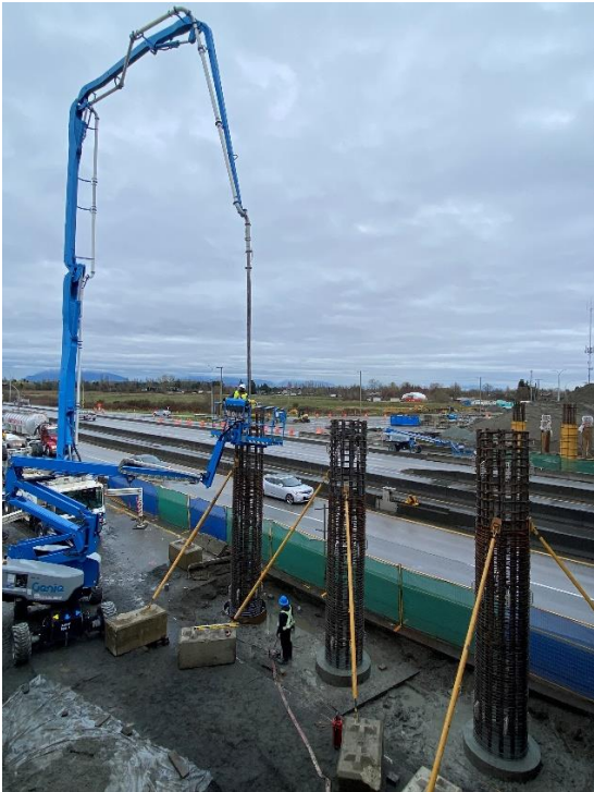
Image 1: Concrete pour through pier column cages
