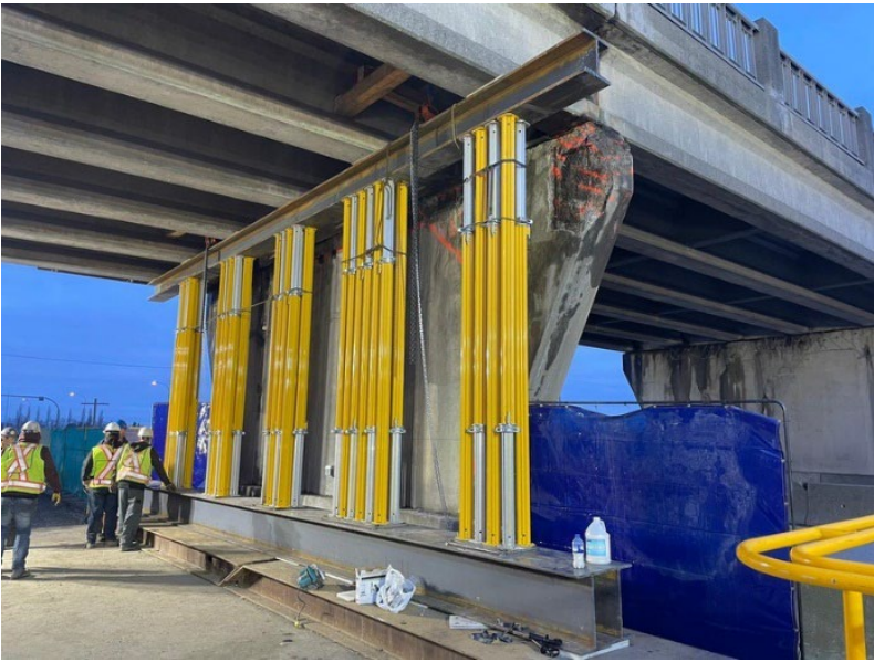
Figure 3: Shoring installed as part of the west pier repair
