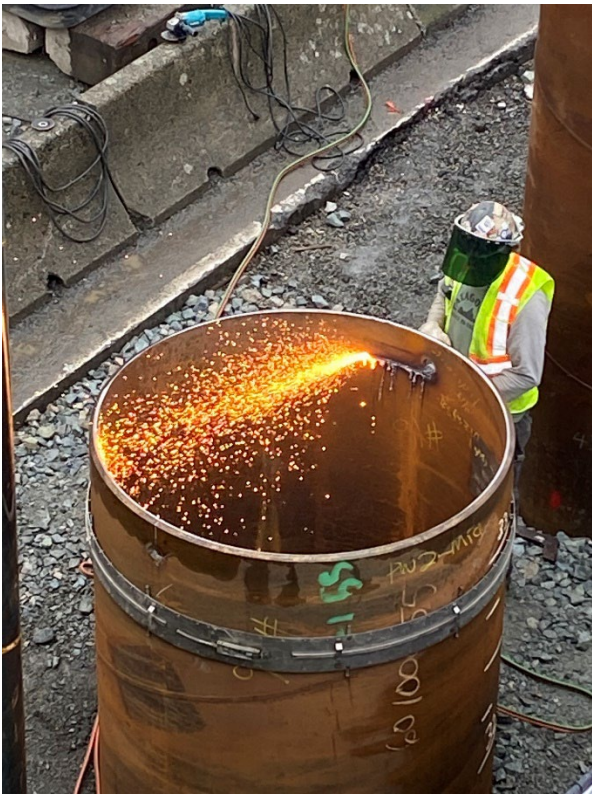
Figure 2: Cutting piles in the northwest quadrant
