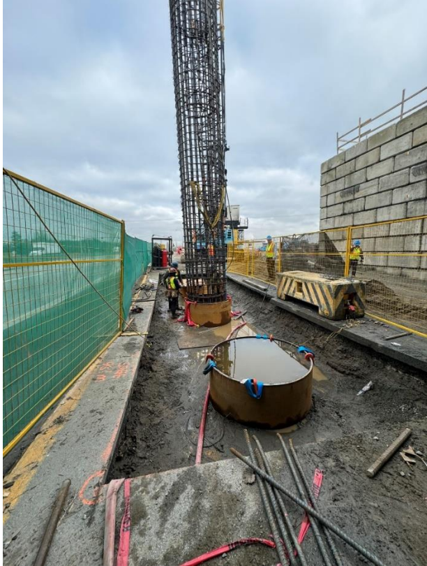
Figure 2: Installing rebar cage
