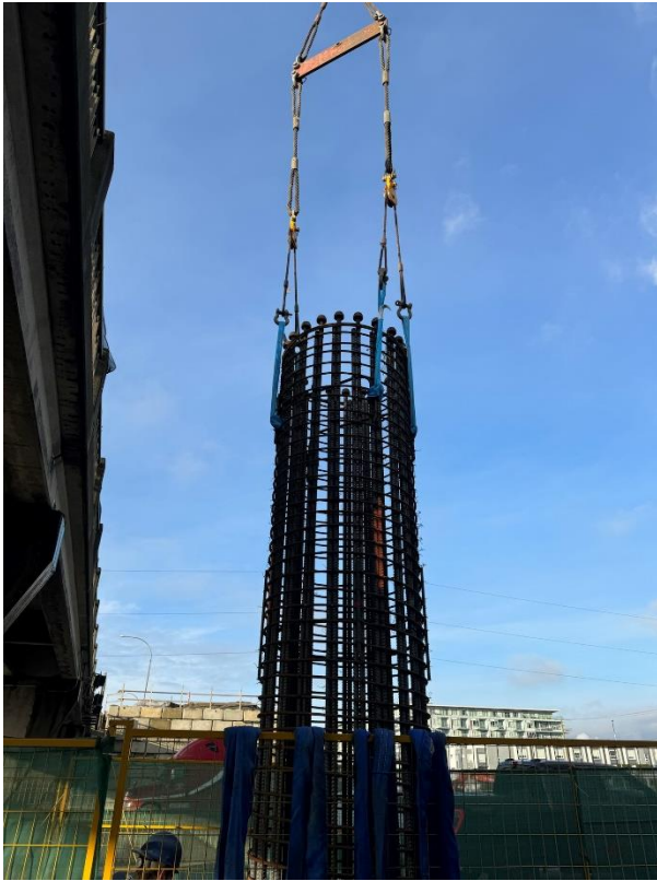
Figure 1: Lifting rebar cage into place
