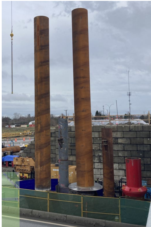
Figure 1 Pier Pile Welding at Northeast Quadrant
