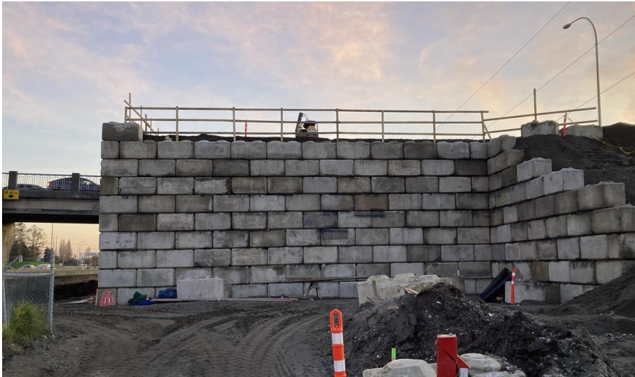
Figure 1 – Temporary Lock Block Wall At Northeast Quadrant
