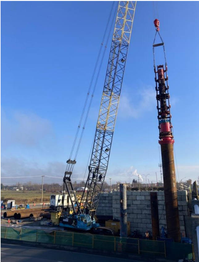
Figure 2 – Pier Pile Driving at Northeast Quadrant
