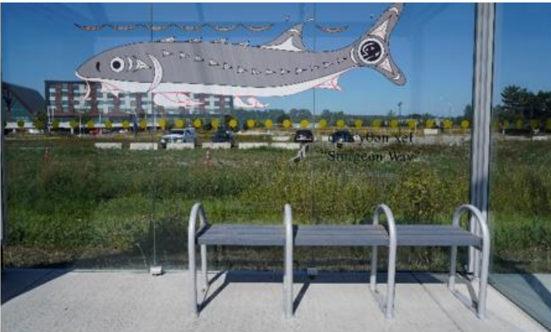
A newly built cycling shelter for people using the bike shuttle to cross the Fraser River.
