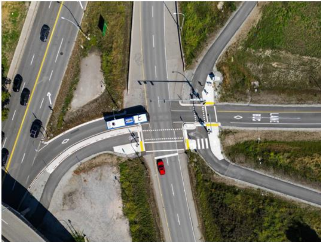
An aerial view of the Bridgeport Road Bus Connection
