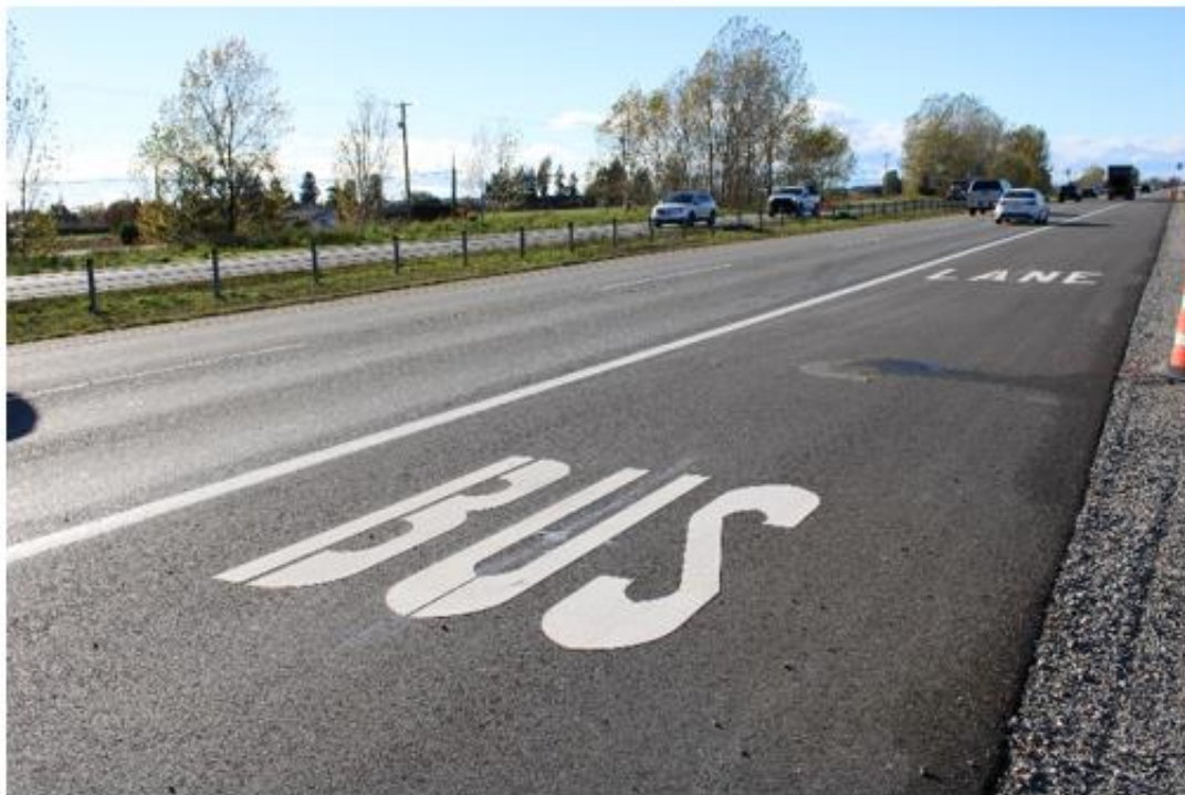
The newly constructed bus-on-shoulder lane on Highway 99 in Fall 2023
