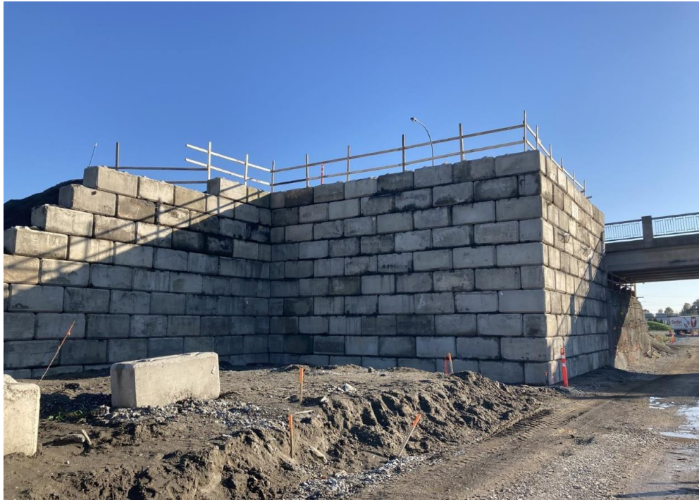
Figure 1 – Temporary Lock Block Wall At Northeast Quadrant
