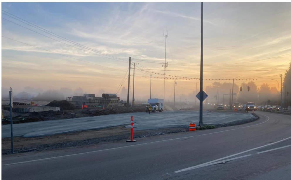
Figure 2 – East Intersection Detour Road Alignment Construction
