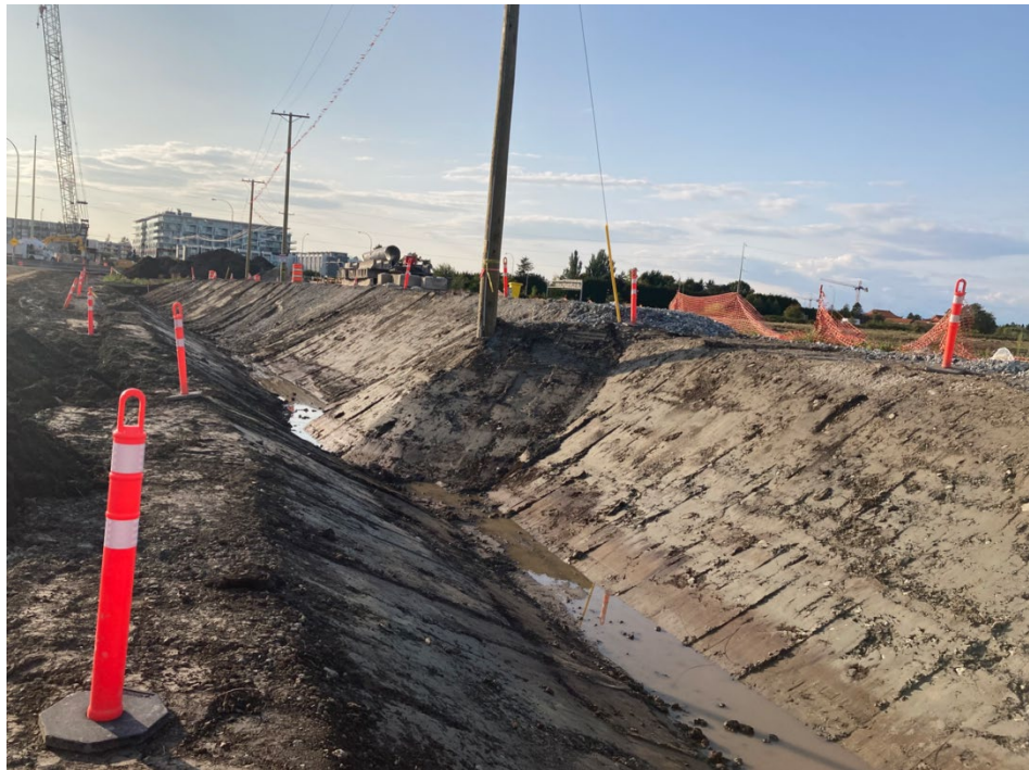
FIGURE 1 – DRAINAGE DITCH CONSTRUCTION AT THE NEW ON-RAMP ALIGNMENT
