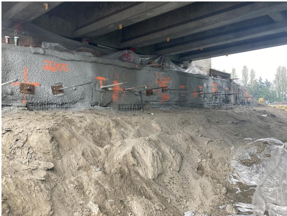
FIGURE 2 – TEMPORARY SOIL NAIL WALL AT EXISTING BRIDGE ABUTMENT
