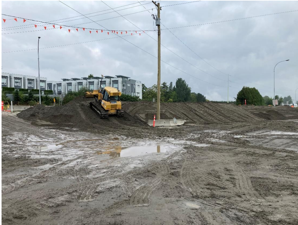
FIGURE 1 – PLACEMENT OF PRELOAD MATERIAL ON THE SOUTHBOUND OFF RAMP
