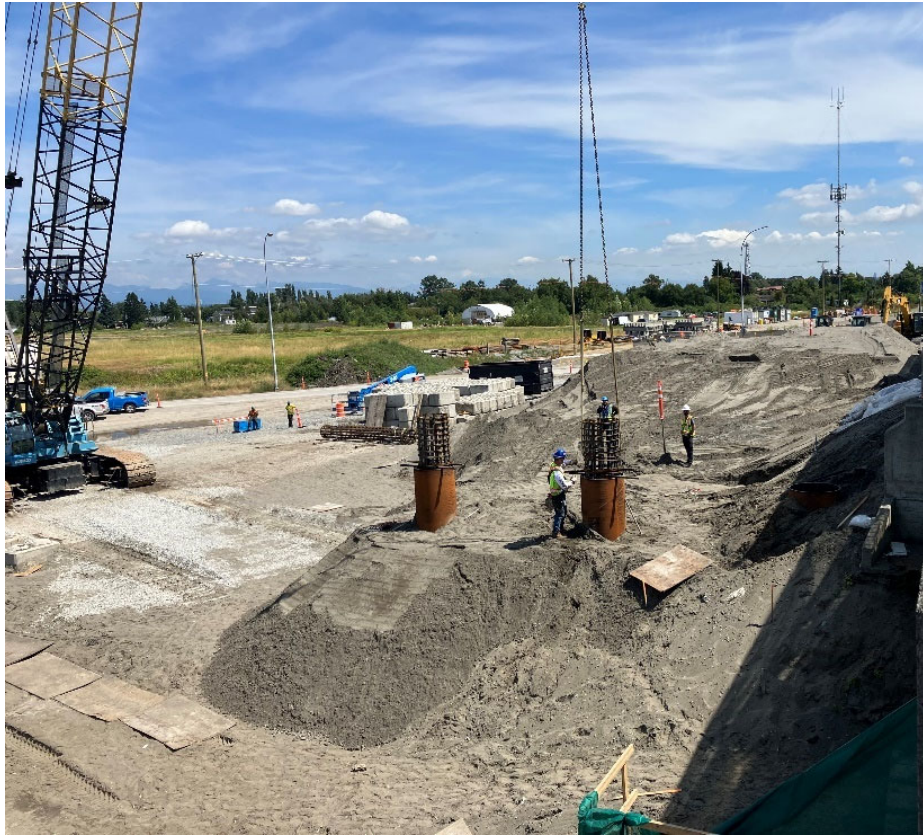
FIGURE 3 – REBAR CAGE INSTALLATION AT EAST ABUTMENT PILES
