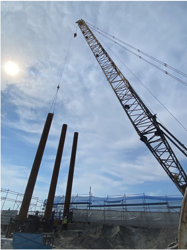
FIGURE 2 – PILE INSTALLATION
