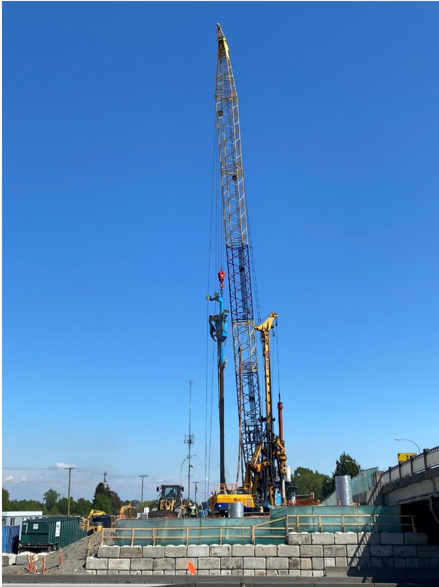
FIGURE 3 – INSTALLATION OF STONE COLUMNS
