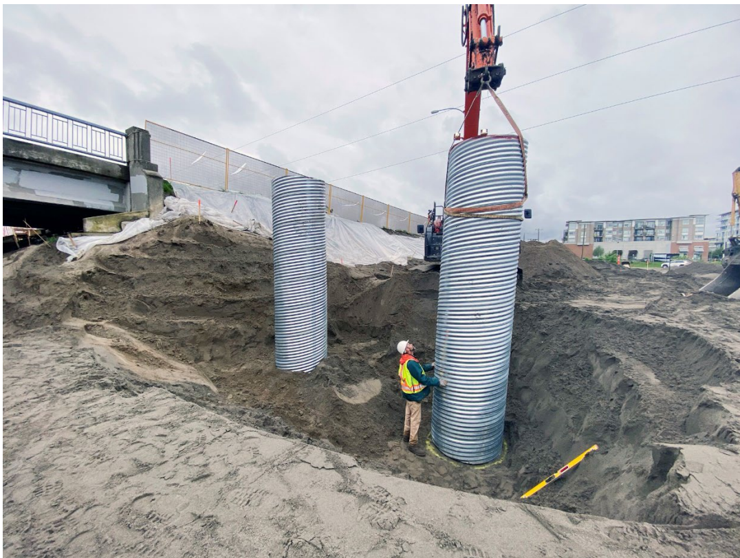
FIGURE 2 – PILE CAISSON INSTALLATION IN THE NORTHWEST QUADRANT (STAGE 1)
