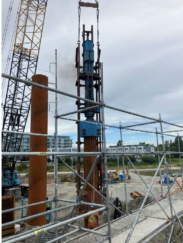
FIGURE 3 – PILE DRIVING IN THE NORTHWEST QUADRANT (STAGE 1)
