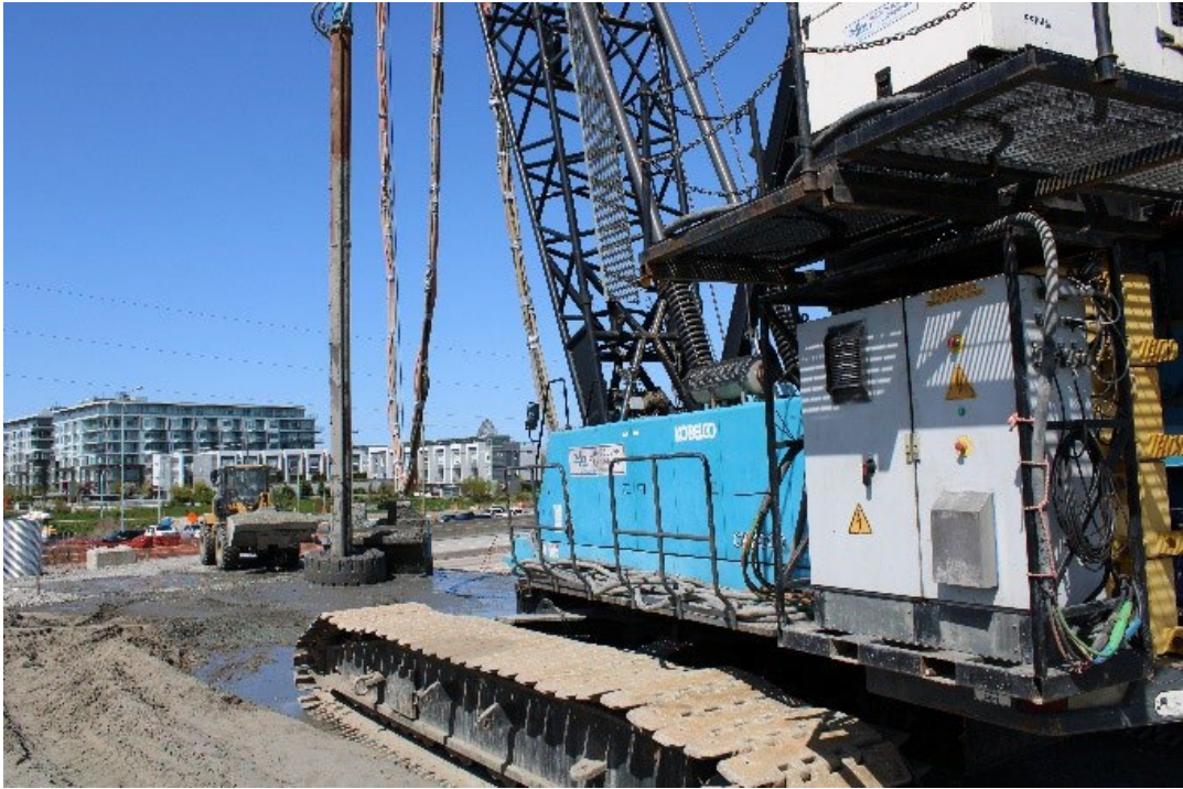
FIGURE 2 – STONE-COLUMN INSTALLATION IN NORTHEAST AREA OF CONSTRUCTION SITE
