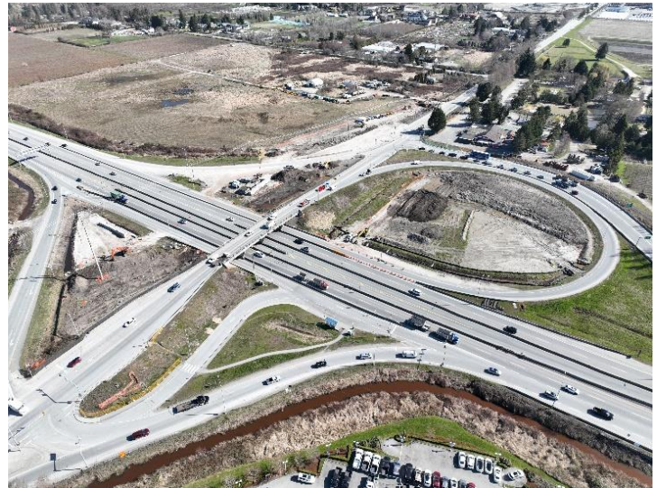
Aerial view of the Steveston Interchange in March 2023 before it is transformed into a five-lane structure.
