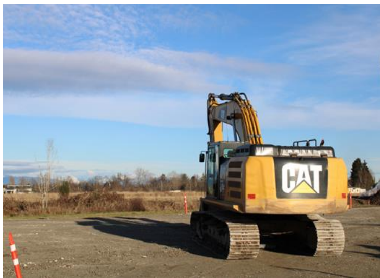
FIGURE 5 – SITE ACCESS CONSTRUCTION
