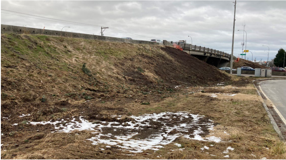
FIGURE 2 – SOUTHWEST QUADRANT POST TREE CLEARING
