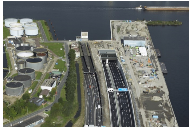
(b) Second Coen Tunnel, Amsterdam, The Netherlands
