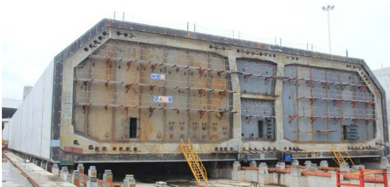
Figure FF Tunnel element being fabricated for the Hong Kong Zhuhai Macao Link in China 63 .
