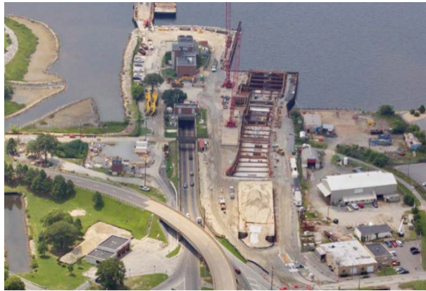
(a) Elizabeth River Tunnels, Norfolk, USA
