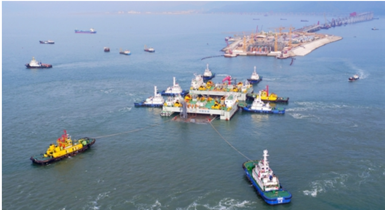
Figure DD Tunnel element being placed in a busy navigable channel for the Hong Kong Zhuhai Macao Link in China 62 .
