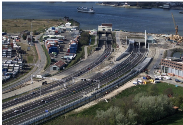
(c) Second Benelux Tunnel, Rotterdam
