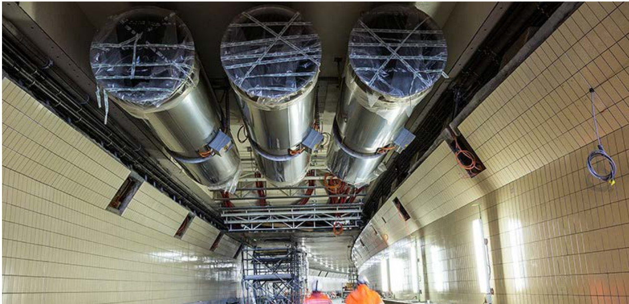
Figure X New mechanical systems that form part of the retrofitting of the Maastunnel currently underway 54 .
