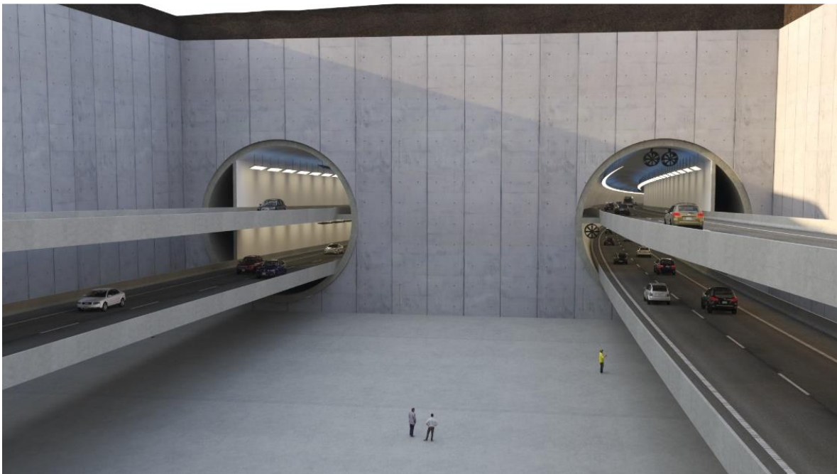
Figure EXEC3: Rendering of the Portal of the Eight-Lane Deep Bored Tunnel Option
