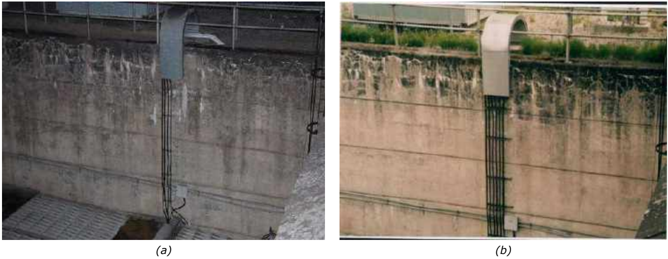
Figure 4-6: Comparison of photo 32 from [1] with (a) showing the condition during the current inspection and (b) the condition during the 2000 inspection – Northern (Lulu) Approach, Element A1, West wall.
