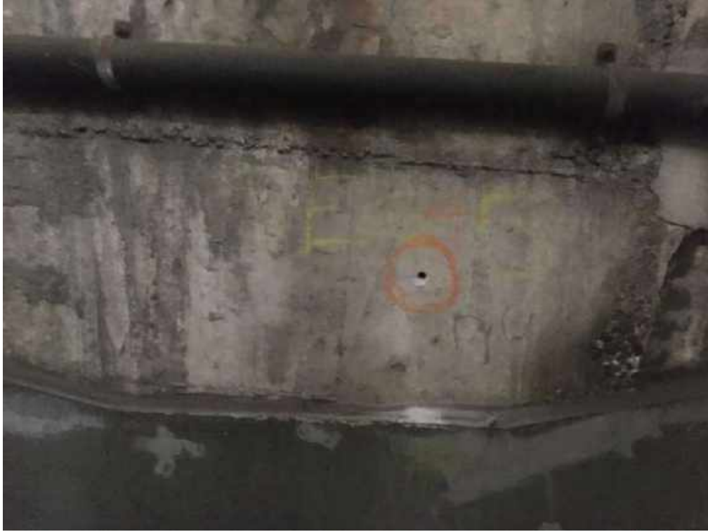
Photo 1 – Typical view of sample location at Downstream Air Duct at Element V/VI at Joint on Outer Wall.
