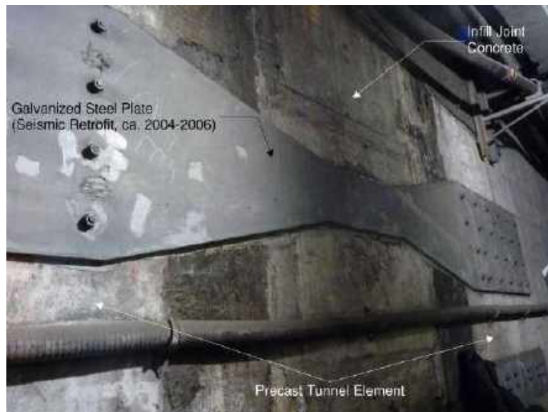
Figure 2-3: Typical example of joint location in outer wall of air duct tubes.
