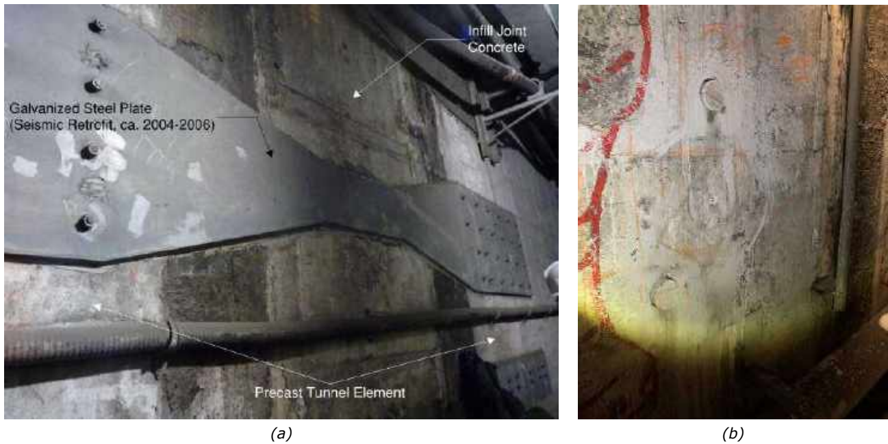
Figure 3-11: Joints between individual immersed tunnel elements as seen in the air duct tubes including at (a) the outer wall (Downstream Air Duct, Joint II/III, Outer wall) and (b) the intermediate wall (Upstream Air Duct, Joint II/III, Intermediate wall).
