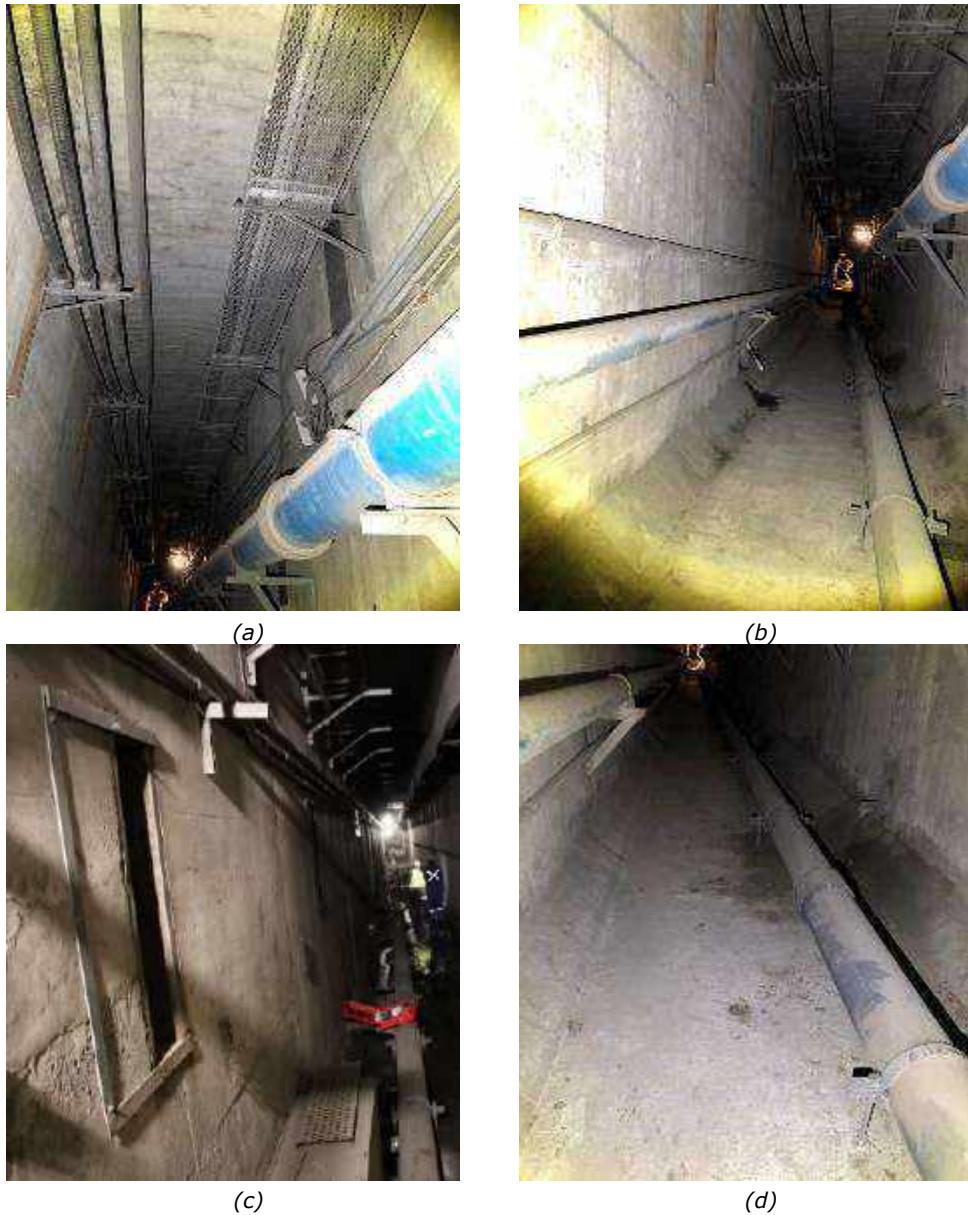
Figure 3-5: Photos of the typical condition of (a) soffit, (b) outer wall, (c) intermediate wall, and (d) floor of the air duct tubes during summer inspection 2020. Dark spots on chamfer and bottom slab seen in (b) and (d) are from water seeping from drainpipes.
