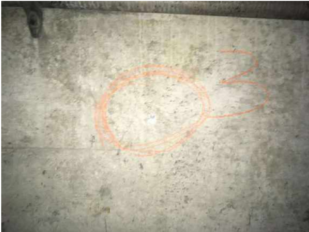
Photo 2 – Typical view of sample location at Downstream Air Duct Element V near 1st Contraction Pour on Outer Wall.
