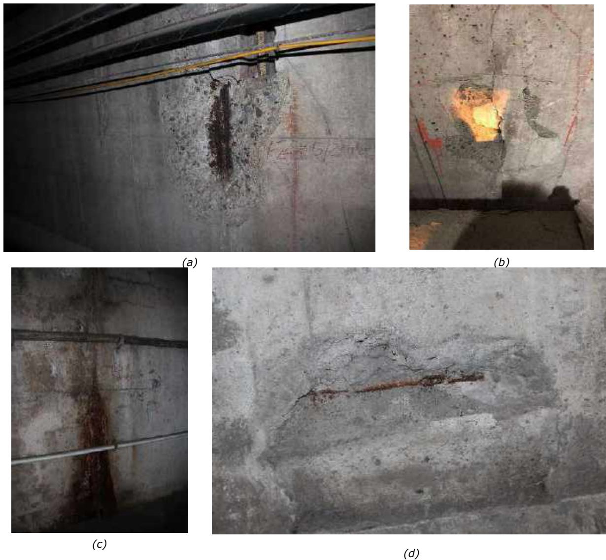
Figure 3-10: Examples of visual signs of reinforcement corrosion including (a) spalling and corrosion staining (Upstream Air Duct, Element IV, Door 22, Outer wall), (b) cracking, delamination and spalling (Downstream Air Duct, Element III, Door 17, Outer wall), (c) corrosion stains on concrete surface (Downstream Air Duct, Element V, Door 29, Outer wall), and (d) spall and exposed reinforcement (Downstream Air Duct, Element II, Intermediate wall).
