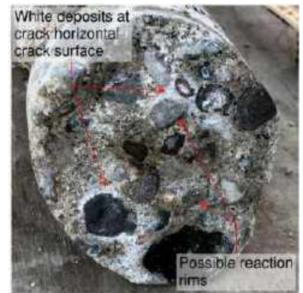
Figure 4-4 Surface of a horizontal crack in Core NAE-P7 from Northern (Lulu) Approach Ramp
